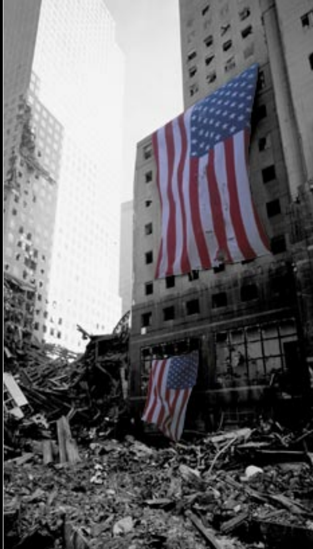
American flags adorn damaged buildings. Photo by Skip Heitzig
