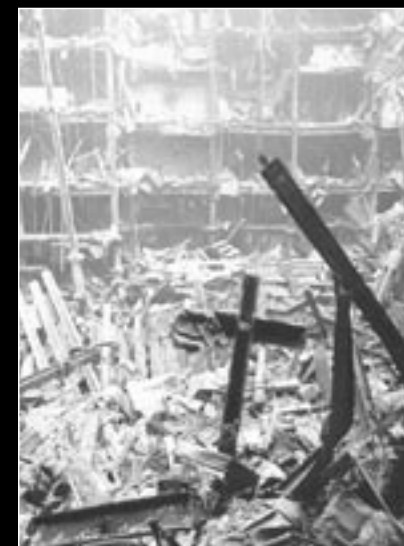
A cross, created in the destruction of the WTC.
